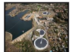
Alvarado Water Treatment Facility - San Diego, CA 1.2 MW System Performing at 115%
